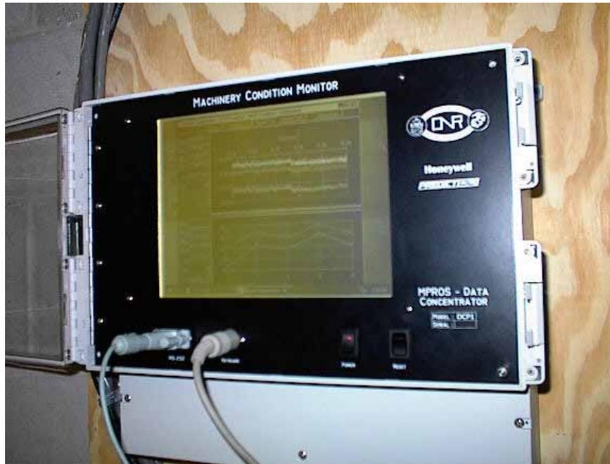
Figure 4. Data Concentrator Installed at HTC
